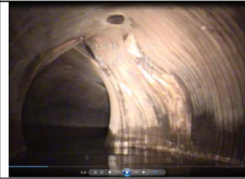
27: Deformation at the Bend Sta. 5 + 25 – 11/9/12
