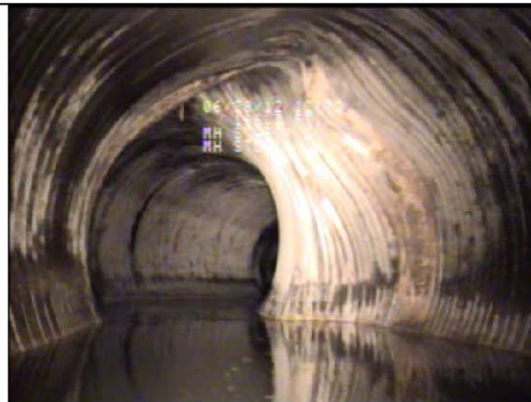
32: Deformation at the Bend Sta. 5 + 33.70 – 6/28/12
